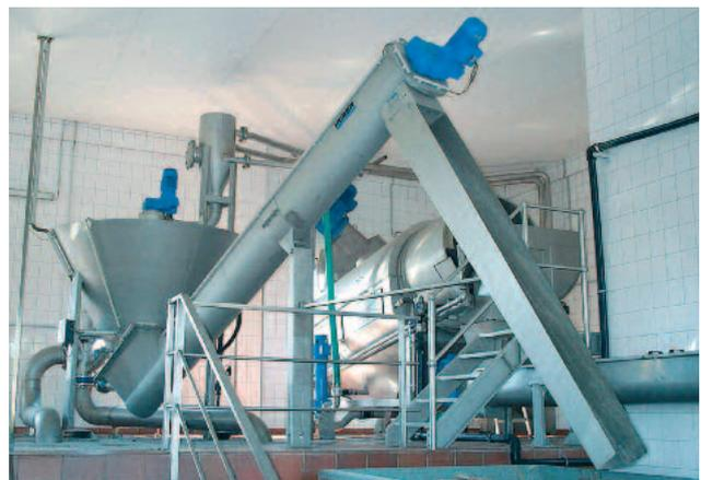
*Wash Drum and Grit Washer installed in the customer's building*
