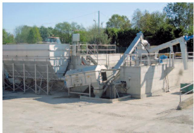
*Acceptance tank for above-ground or underground installation*
