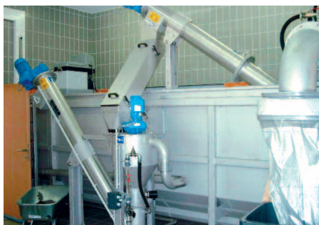
Classifying screw with subsequent HUBER Coanda Grit Washer RoSF4 TC
