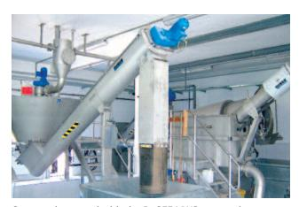
Sewer grit treated with the RoSF5 VWS system is recycling material.
