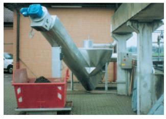
HUBER Coanda Grit Classifier RoSF3 installed subsequent to a grit channel
