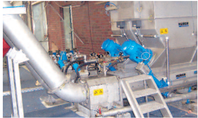
The HUBER Screenings Wash Press WAP® SL HP for optimal screenings treatment
