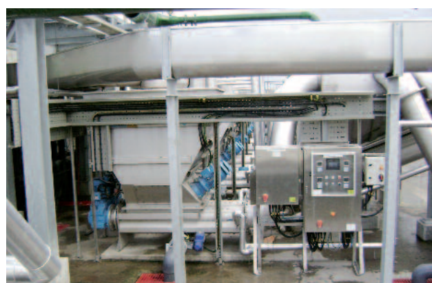
WWTP Dublin (Ireland): 2 million PE HUBER Launder Channel: 30 m 3 wastewater per second
