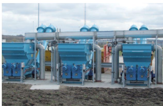
WWTP Knostrop (UK): 2 million PE HUBER Launder Channel: 20 m 3 wastewater per second
