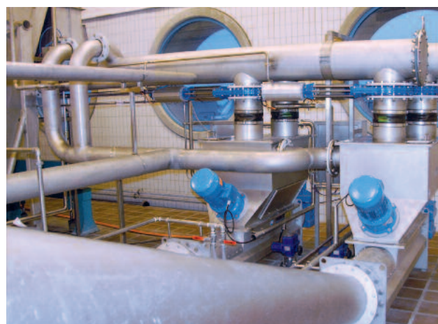
HUBER Launder Channel system feeding redundant HUBER Wash Press WAP/SL units
