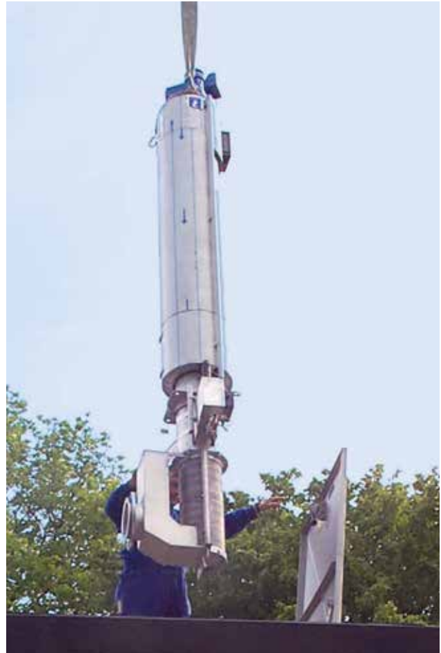
HUBER Pumping Stations Screen ROTAMAT® RoK4 being lifted into a pumping station.
