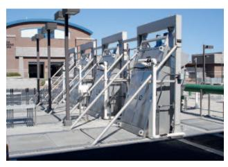
4 HUBER Fine Screen STEP SCREEN® SSV units: L= 5300, W=1376, 6 mm slot width, installation angle 75°. Maximum operational stability due to the special bottom step design for increased operational reliability without impairment by grit, gravel, stones.
