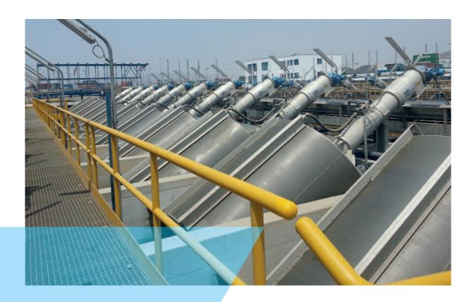
Reliable and well-proven inlet screen for municipal sewage treatment plants and industrial wastewater and process water screening
