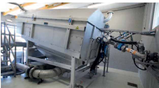
HUBER Sludge Acceptance Plant RoFAS with metering system for pH and conductivity measurement
